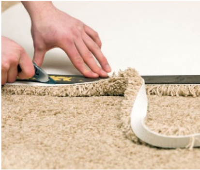
Installation off - cuts
